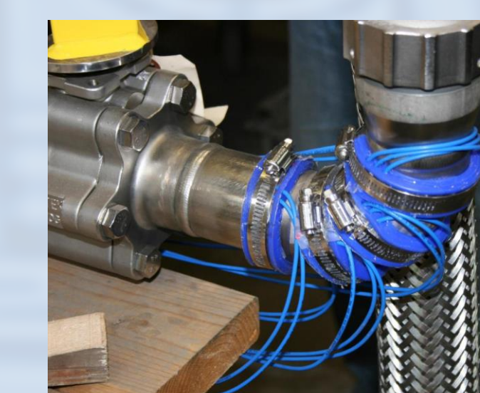
Figure 14. Installed Pipe Wrap™
