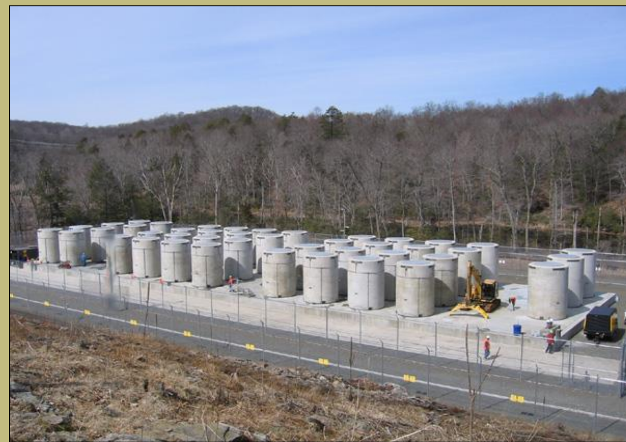
Figure 1: Connecticut Yankee dry storage site [2]
