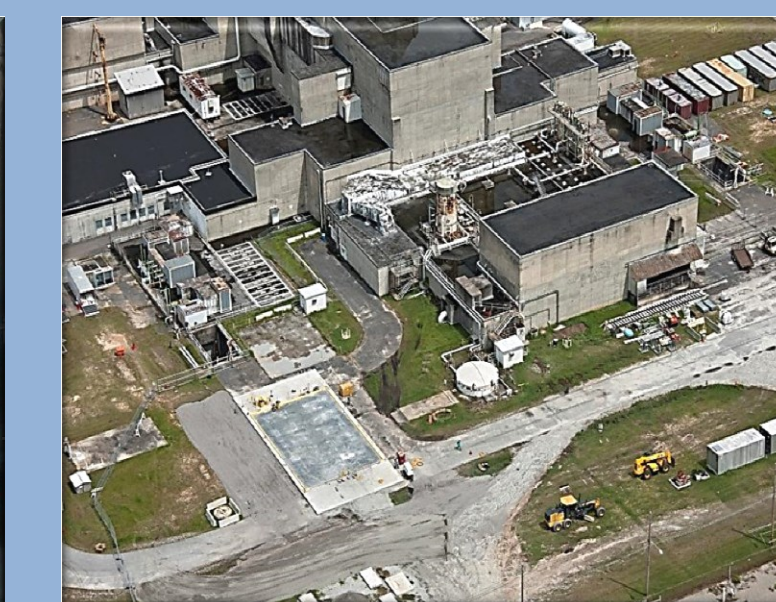
105-C Site After Final Clean-up
