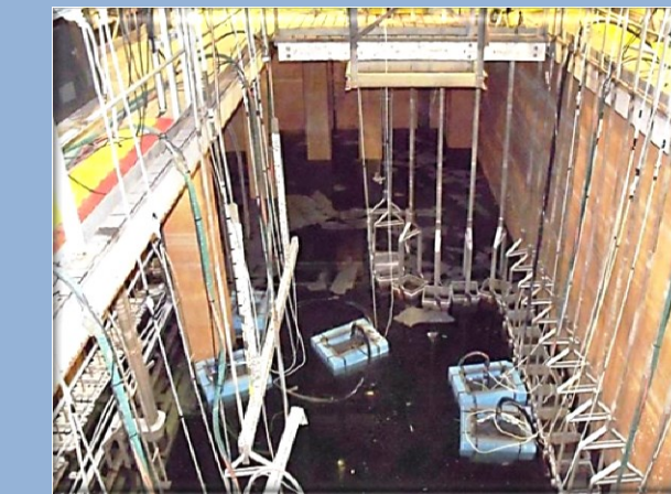
Machine Basin at -4.88 meter level
