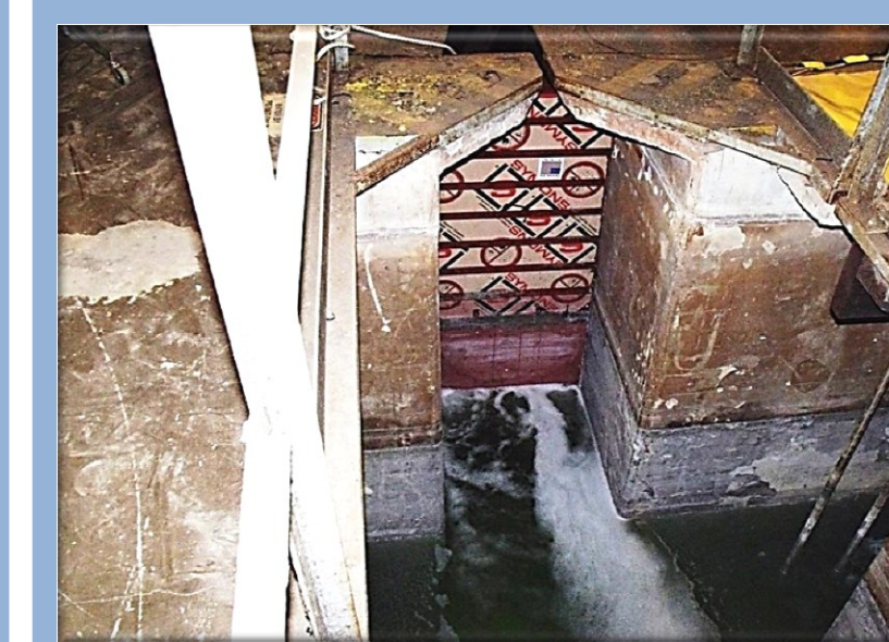
Installed underwater grout to -4.88 meter level
