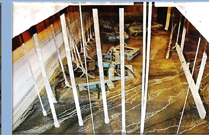
Encasing floatation devices in Machine Basin in grout
