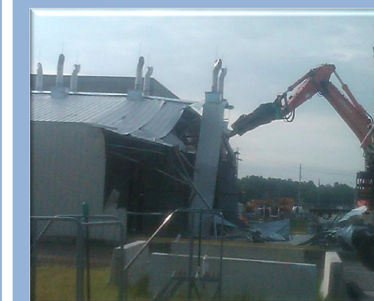
Demolish Evaporator Shelter
