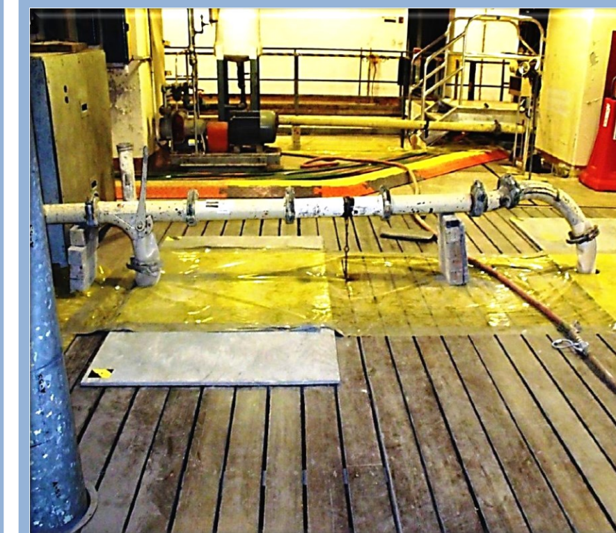
Machine Basin During Grouting
