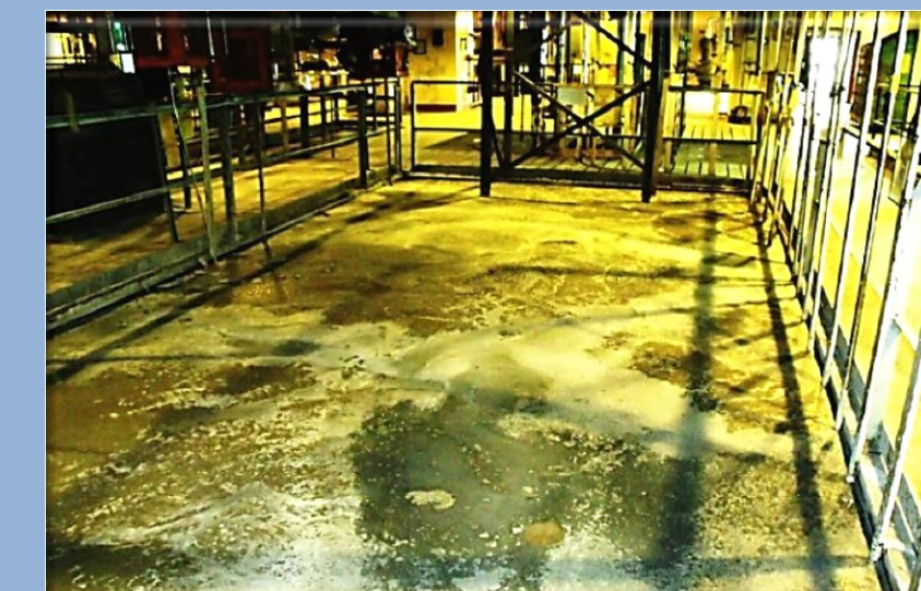
Machine Basin After Final Grout Lift
