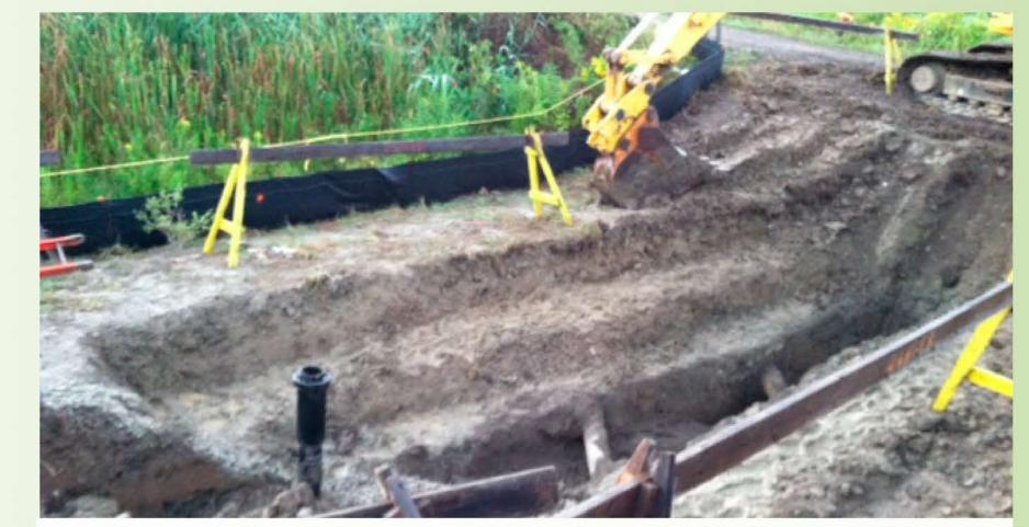
\* Abandoned Oil Lines and Contamination **Encountered During Pad Excavation**
