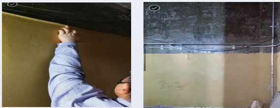
Figure 2. Coated wall to the height that workers can reach
