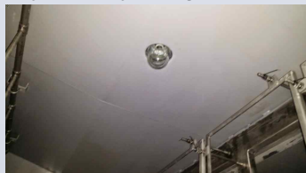
Figure 3. Interior lights that can be replaced from outside ceilings
