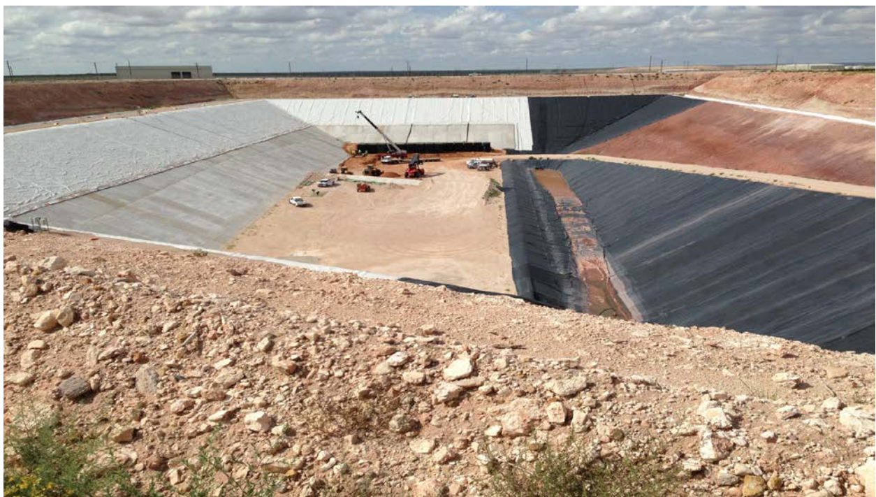
Fig. 2. WCS Federal Waste Disposal Facility
