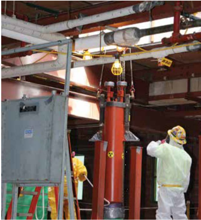
Fig. 5. Safe removal of a NaF trap used in the K-27 Building.
