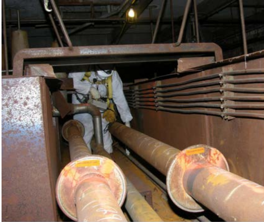
Fig. 3. A worker performs non-destructive assay work inside K-27.
