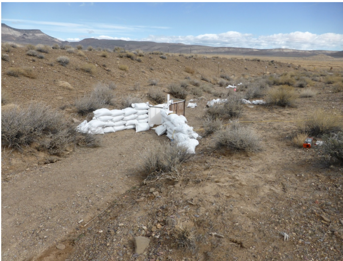
Figure 5. View looking downstream at the flume installed in a channel on the Smoky Site. A pressure transducer (used to measure flow depth) is installed at the flume, and the data are transferred to an environmental monitoring station located just off of the right edge of the photo.
