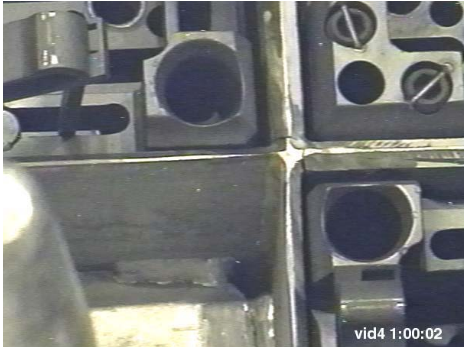
Fig 11. Weld Location #1--1999 Inspection (INEEL/EXT-01000183, 2001)
