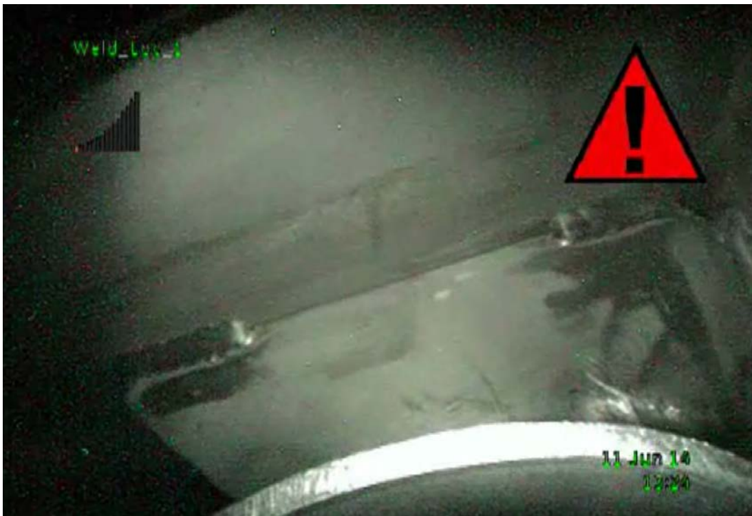
Fig 7. Photo from 2014 Inspection
