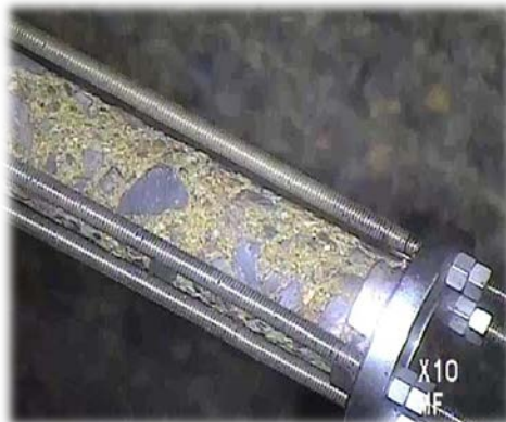
Fig. 17. Concrete Corrosion Coupon Inspection
