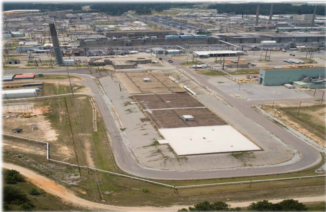
Fig. 2. H-Canyon Sand Filter Facility
