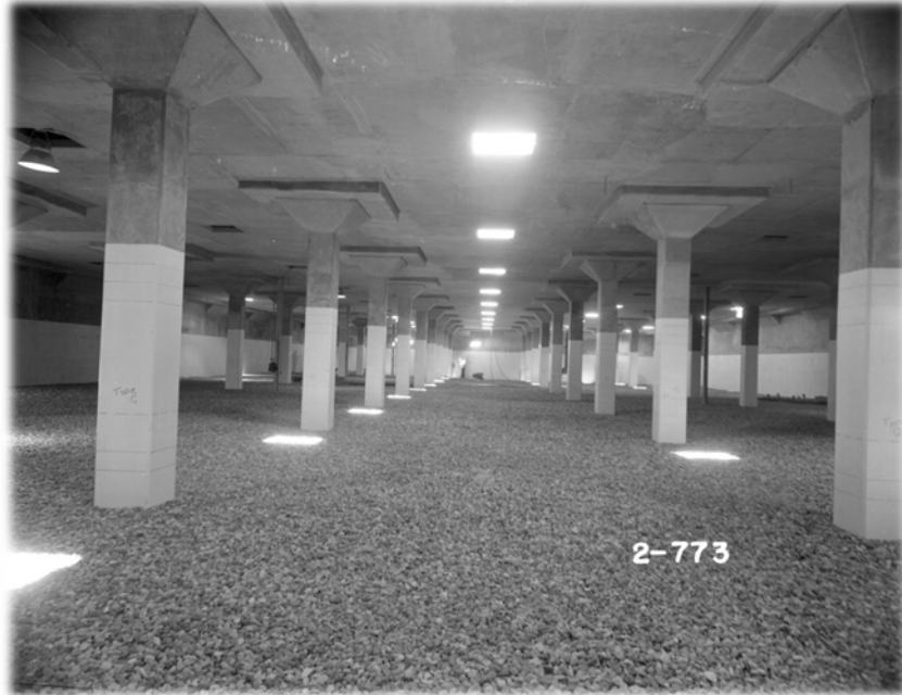
Fig. 3. Original Sand Filter/Tunnel Internal Construction
