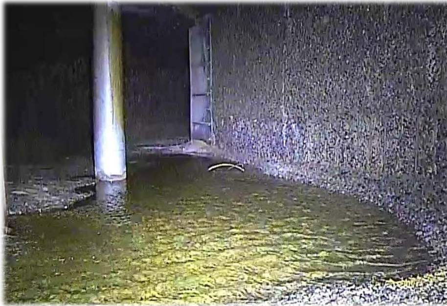
Fig. 16. Tunnel Conditions, After Pumping
