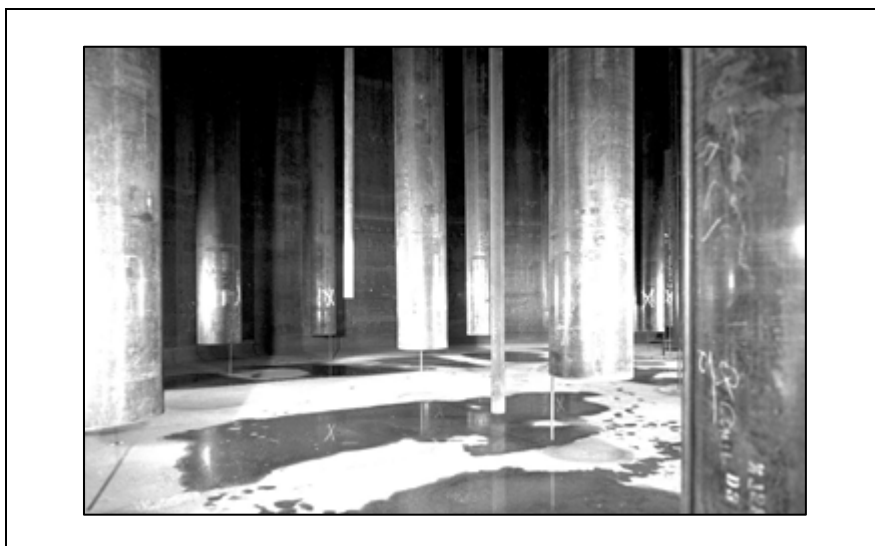
Fig. 5. Tank AY-102 Interior with Airlift Circulators
