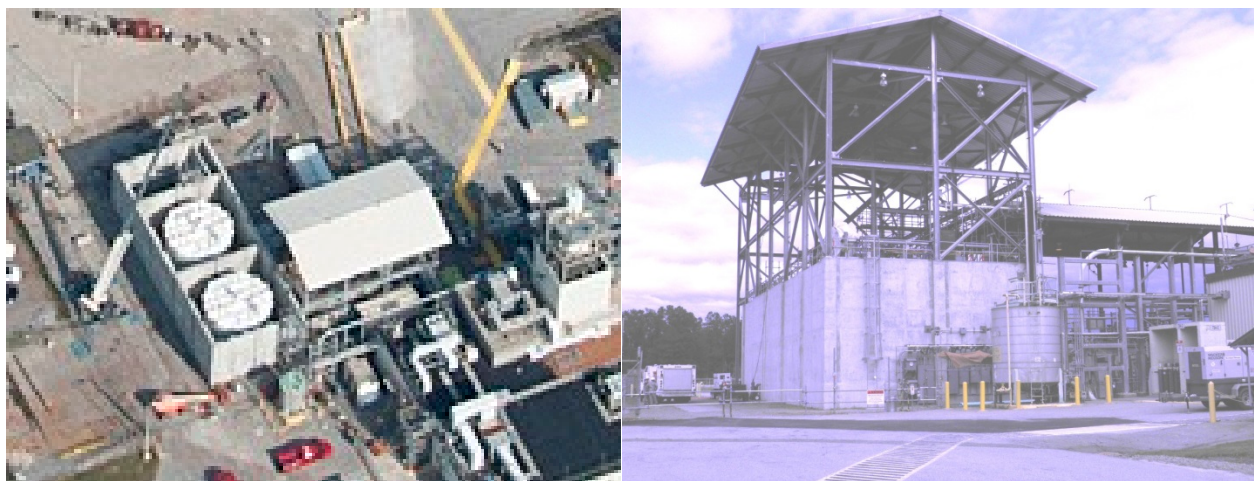
Figure 3. Salt Solution Receipt Tanks
