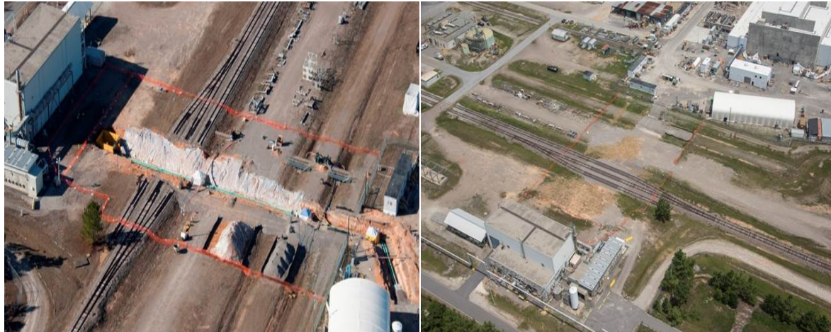
Figure 7. Installation of West Transfer Lines
