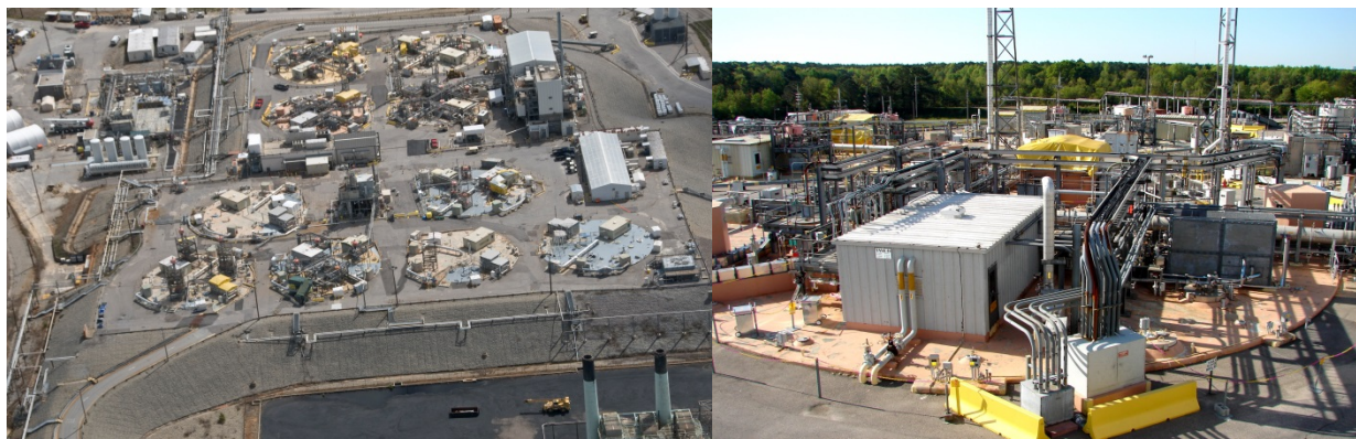
Figure 5. Tank 49H – Future Feed Tank for SWPF
