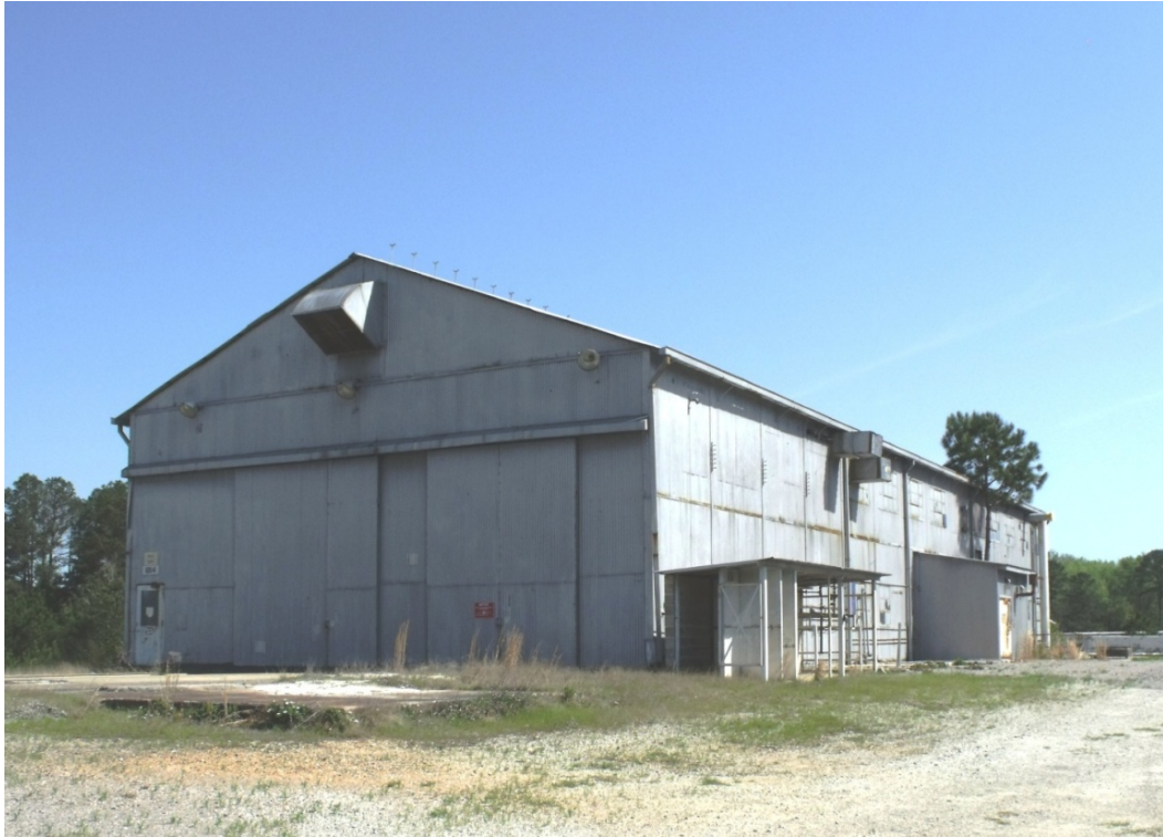
Photo 1: 690-N (Ford Building) - Looking Northeast
