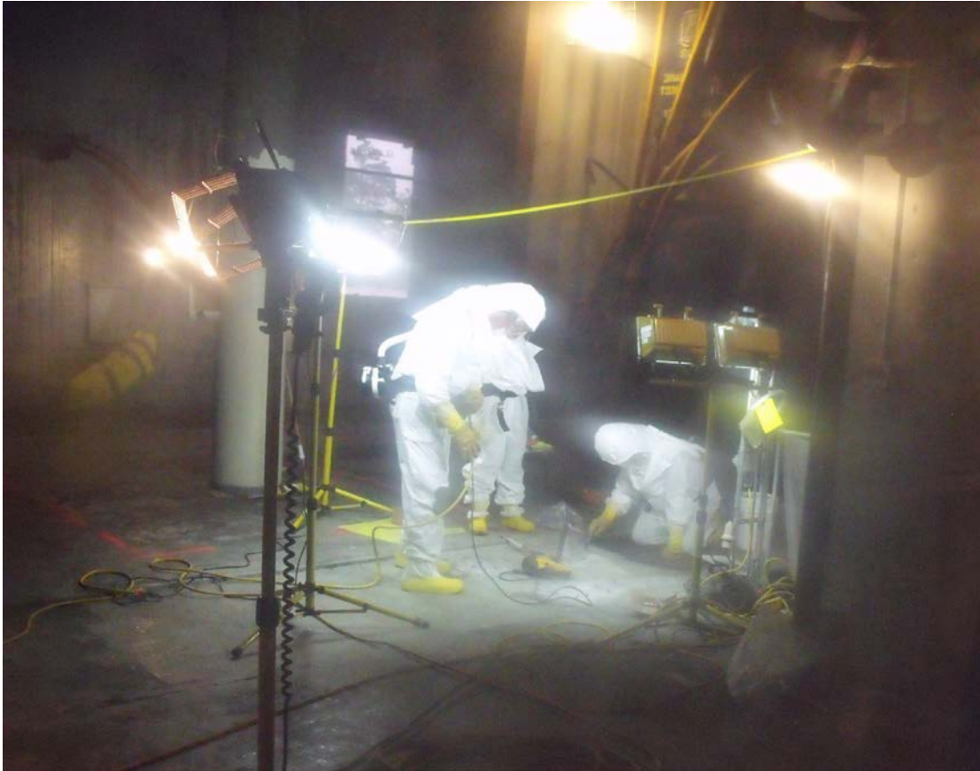
Photo 2 – Concrete Floor Sampling
