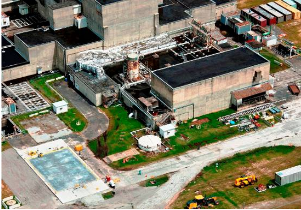
Fig. 3 – Basin Segment After Grouting
