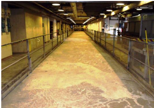
Fig. 2 – Building 710-C After
