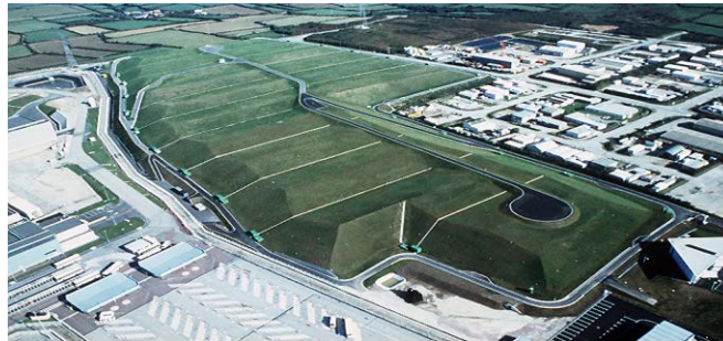
Figure 6: general view of the facility after closure
