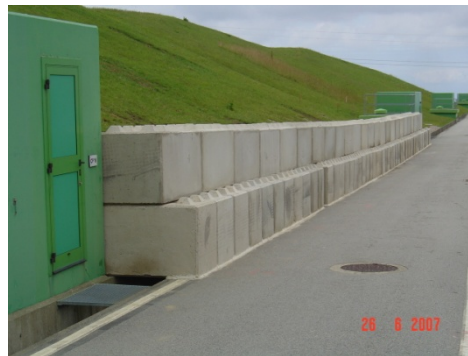
Figure 8: reinforcement of the slope of the capping system
