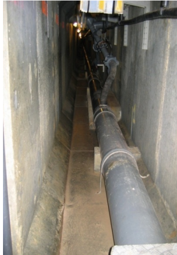
Figure 4: implementation of the monitoring gallery
