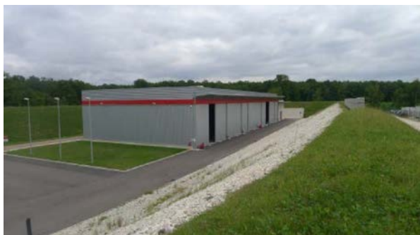
Figure 7: storage facility for institutional wastes
