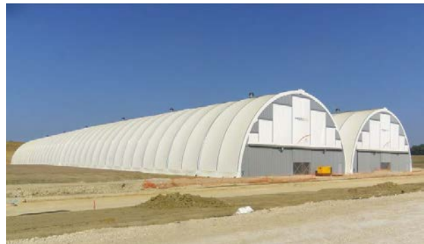
Figure 4: the move of mobile roof is presently performed using cranes (on the left). Rails will be used for the move of sections of the new mobile roofs (on the right, Premorail®)
