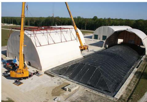
Figure 4: the move of mobile roof is presently performed using cranes (on the left). Rails will be used for the move of sections of the new mobile roofs (on the right, Premorail®)
