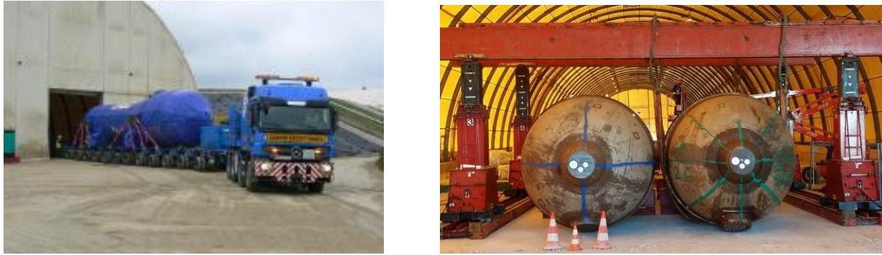
Figure 6 : disposal of steam generators
