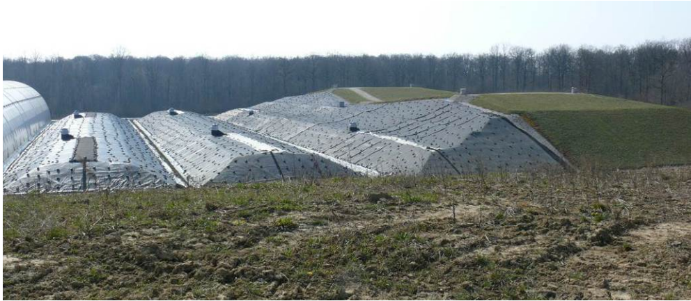
Figure 5: implementation of the capping system
