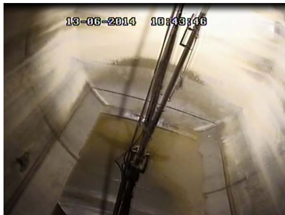
Fig.7: Final state of the tank after the emptying operations
