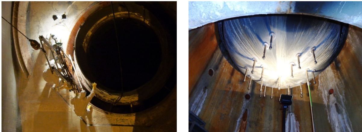
Fig. 5. Cutting of primary piping (left) RV bottom with insulation removed (right)
