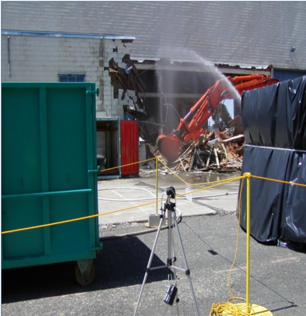
Fig. 4 Perimeter Sampling During ACM D4 Activities
