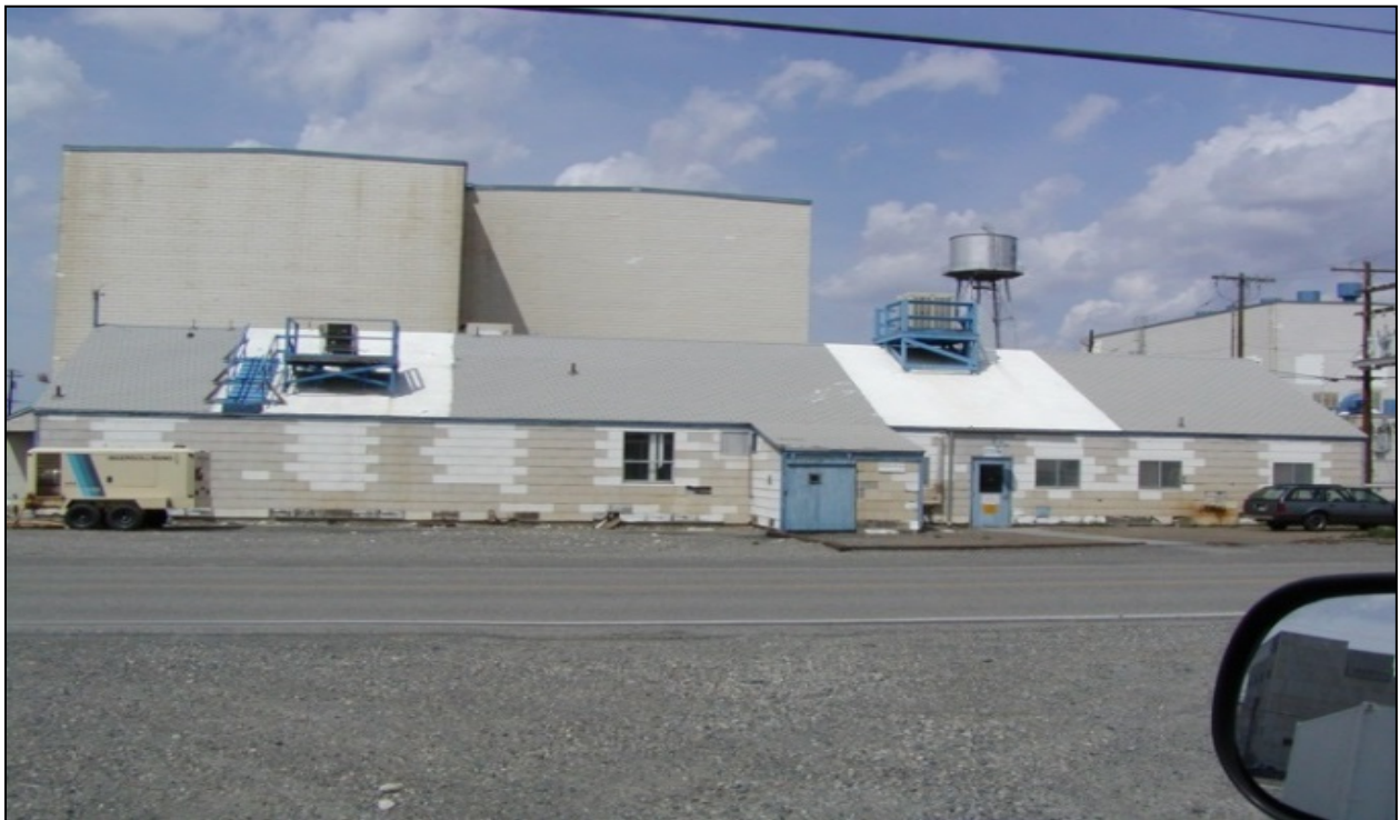
Fig. 2 Transite-Sided Building in the Hanford Central Plateau Area
