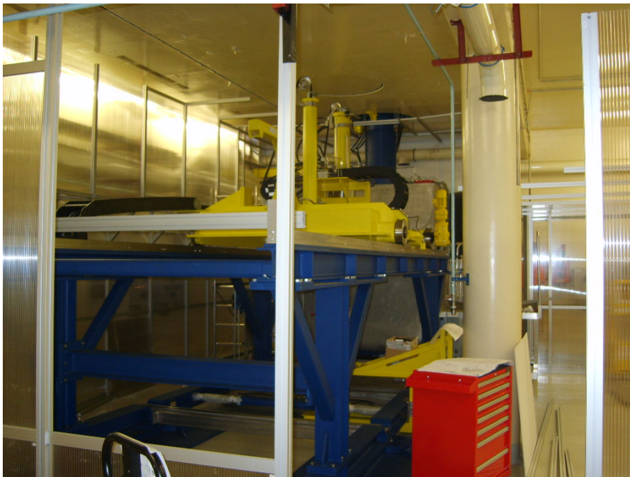
Fig.6: Equipment set-up in the BCOT vault
