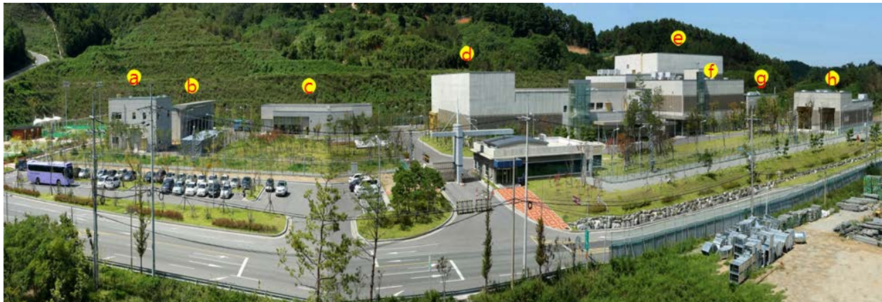
Fig. 3. Layout of the Wolsong LILW surface facilities ; a) Waste water treatment building, b)Garage, c)Equipment maintenance shop & warehouse, d)Radioactive waste receipt & storage building, e)Radioactive waste treatment building, f)Service building I, g)Service building II, h)Power supply building
