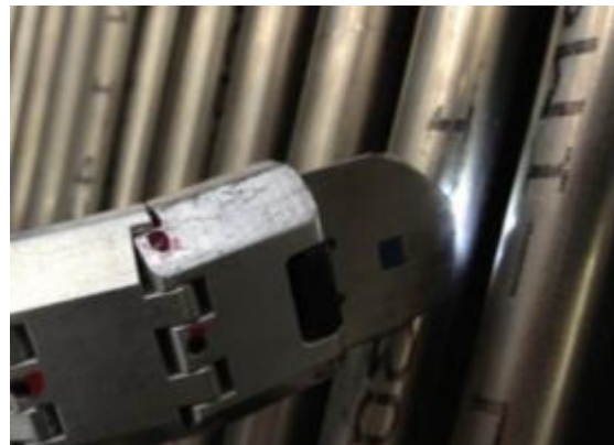
Fig. 11 – Service equipment - BICS
