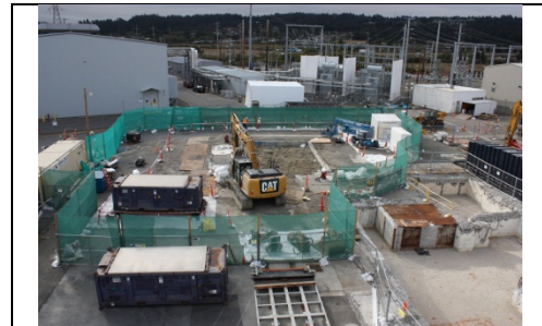
First demolition - Hot Machine Shop
