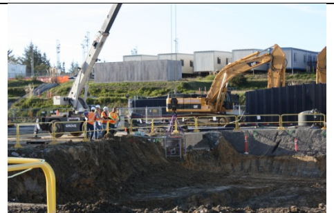
Pre-trenching water cut-off wall
