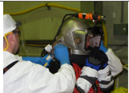
Divers removing spent fuel pool liner wet
