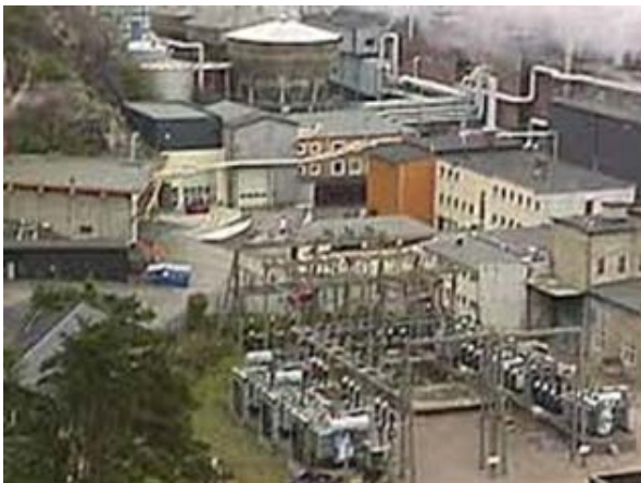
Fig. 2. The Halden site with the entrance to the underground facility to the left.
