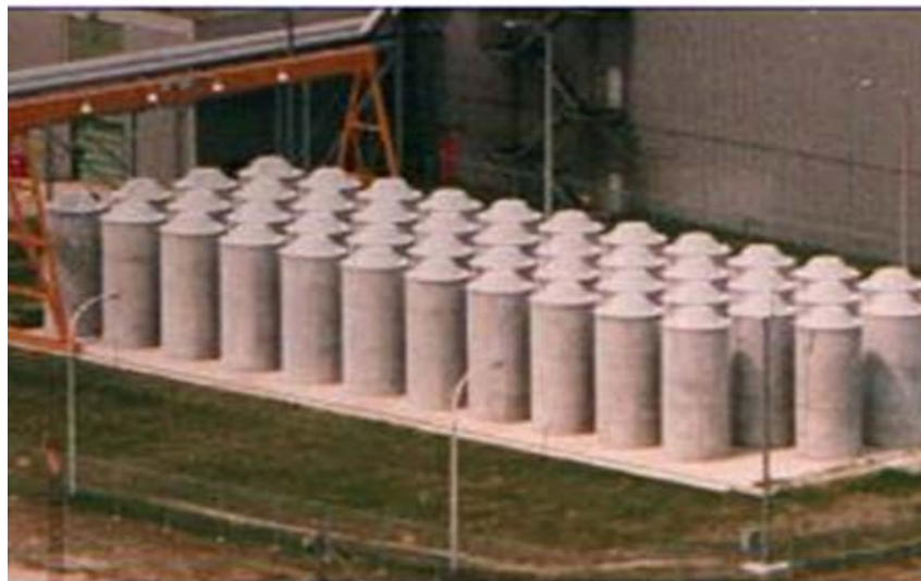
Figure 3 – Concrete Canisters at Douglas Point Decommissioned Facility
