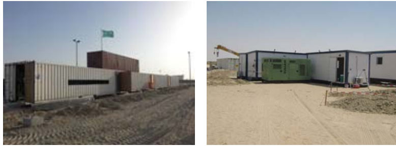
Picture 1, 2: Site with containers for decontamination plant
