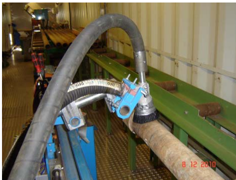
Picture 13: outer surface cleaning of pipes
