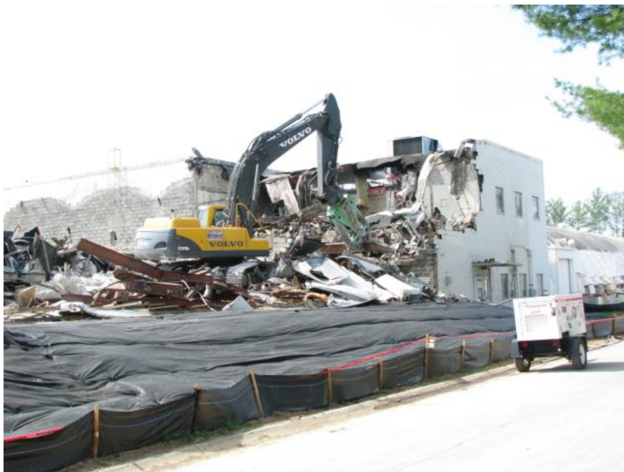
Fig. 2. Building 2024 demolition using a trackhoe with an attached shear.
