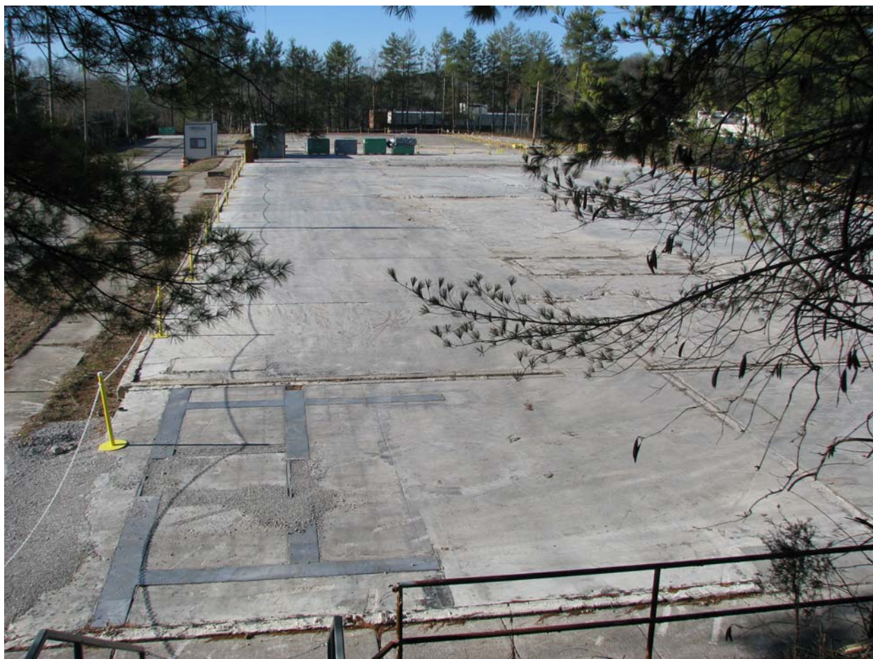
Fig. 3. 2000 Complex slabs following demolition.
