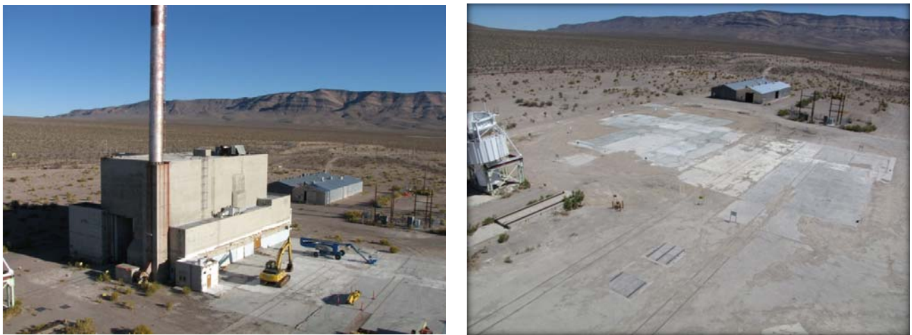
Fig. 1. Before and after photos of the R-MAD Facility.
