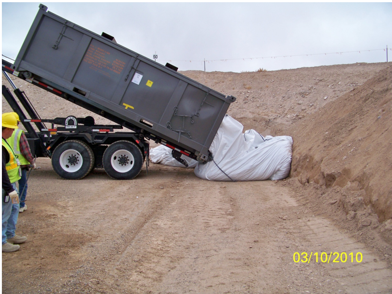
Fig. 2. Picture of first R-MAD intermodal offload at Area 5, Disposal Cell 17.
