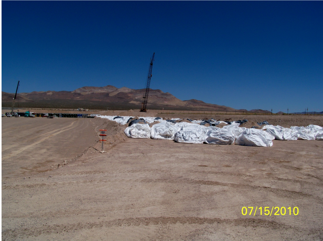
Fig. 3. Cell 17 placement of R-MAD intermodal debris.
