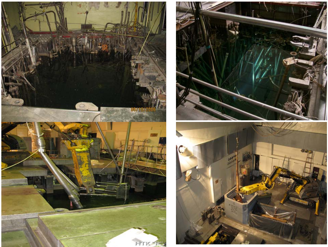
Fig. 3. Removal of loop channels from the reactor pool.
