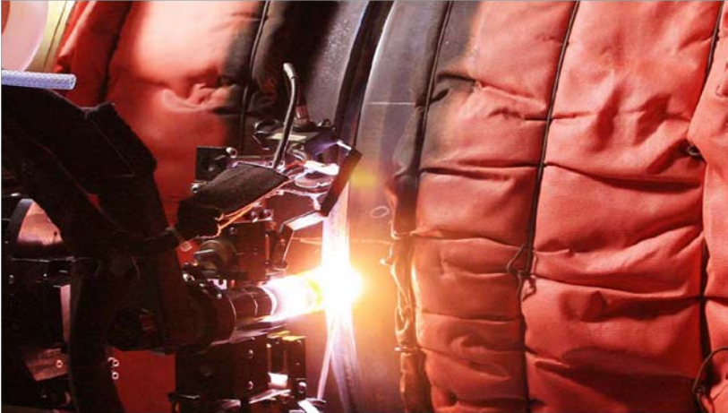
Automatic Welding Machine -Shin-Kori
