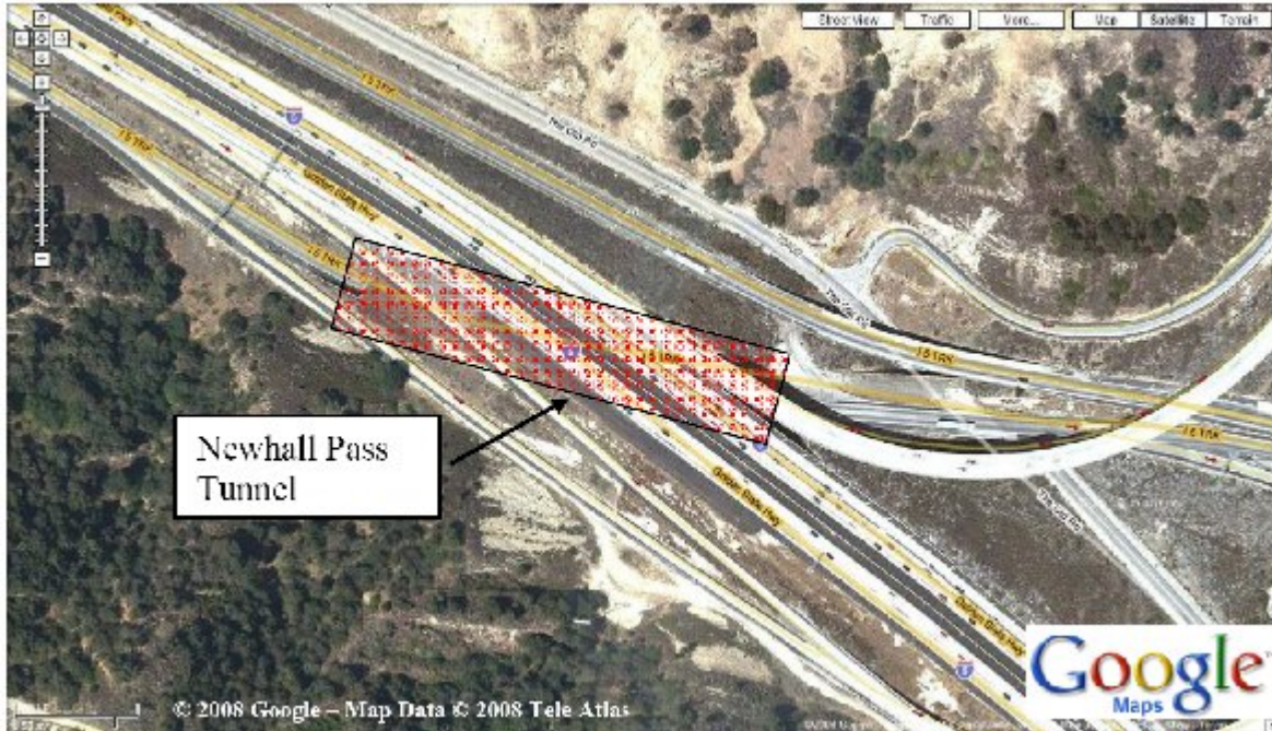
Fig. 5. Aerial Photograph of Interstate 5 and Highway 14 Interchange. The Accident Initiated on the Exit (Southwest Side) of the Tunnel.
