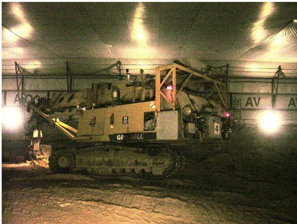
Fig. 4. Buried waste exhumation operations in the Accelerated Retrieval Project III, Pit 6.
