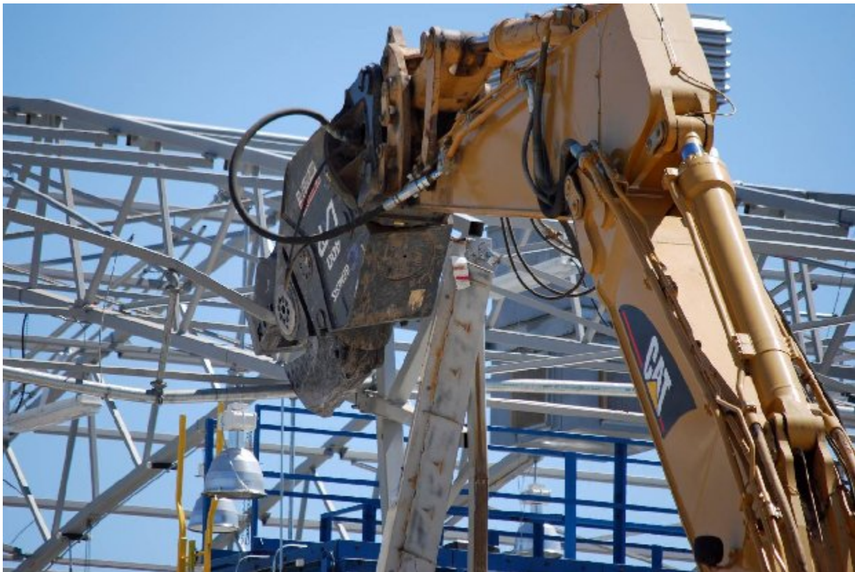
Fig. 3. D&D of the Excavator Method Project facility (WMF-671).
