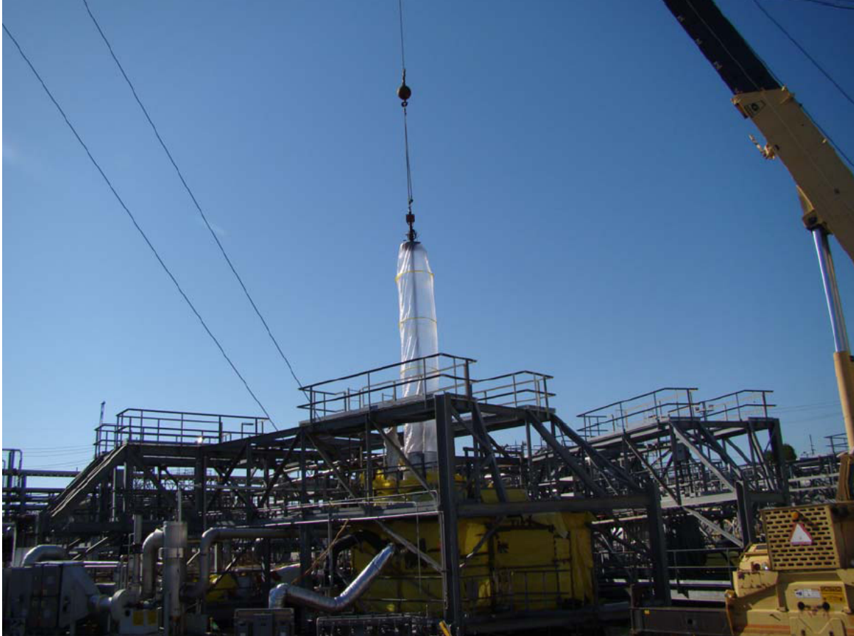
Figure 1: Installation of Sampler and Mast Assembly in an SRS Waste Tank
