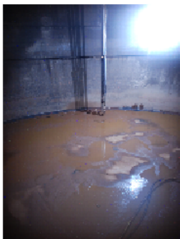
Tank 19 wall and floor
