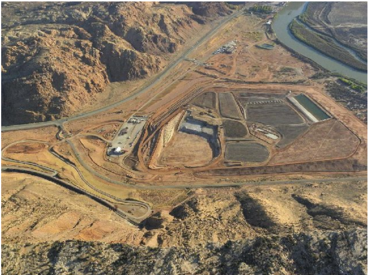
Figure 1. Aerial view of Moab Site looking east.
