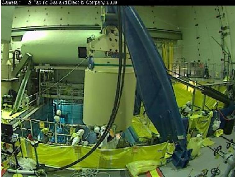
**Figure 9 - Davit Crane Lowering HI-STAR HB into SFP**
