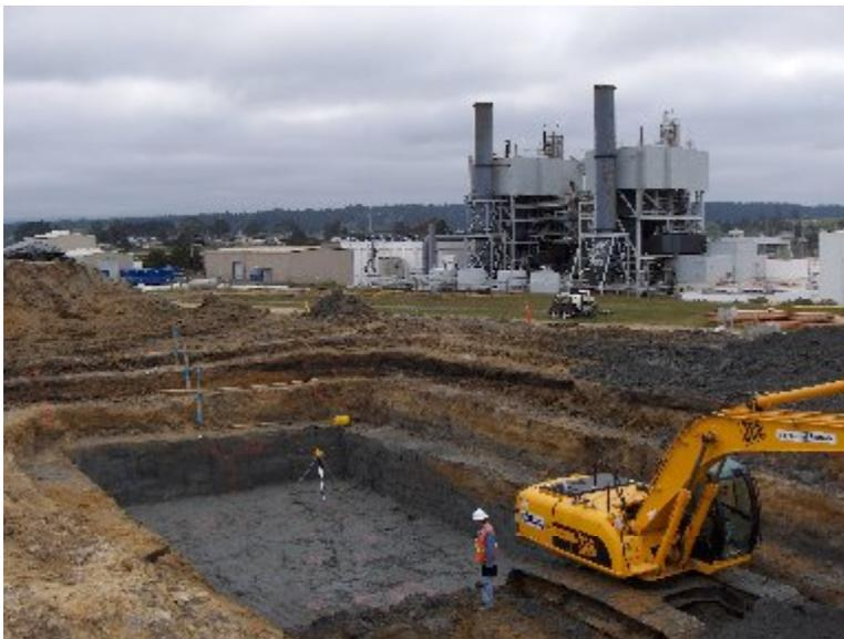
**Figure 6 - Excavation for ISFSI Vault**
