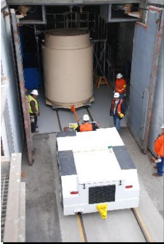
**Figure 15 – Removing a Loaded HI-STAR HB from the Refueling Building Using the Airplane Tugger**
