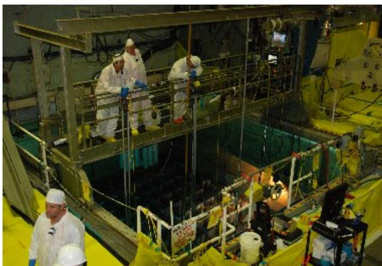
**Figure 12 - Loading Fuel into an MPC**
