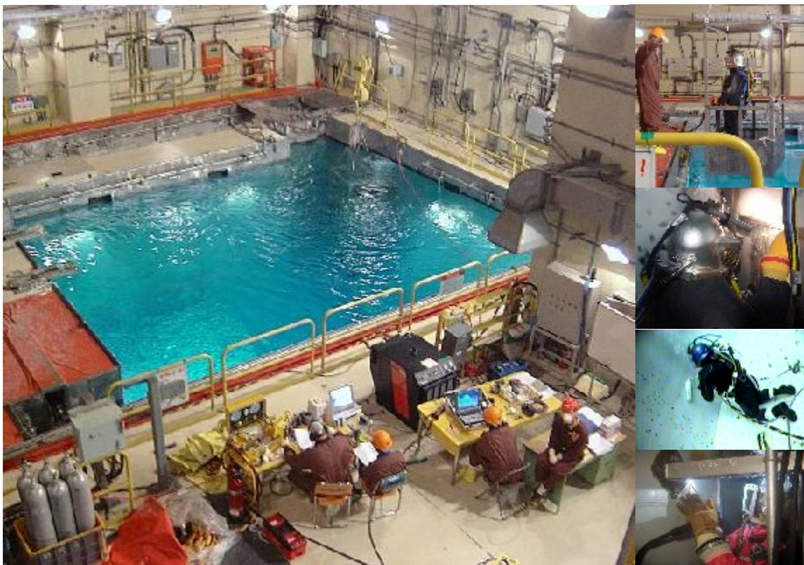
Fig. 1. Typical diving operation. Clockwise from left: dive control station, diver entering fuel pool, diver inspector, diver applying fixative, and diver welding.
