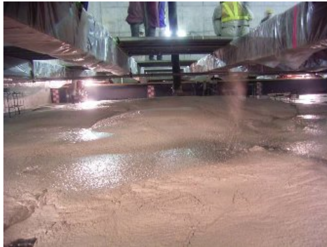
Fig. 14 Mortar placed directly on bentonite
