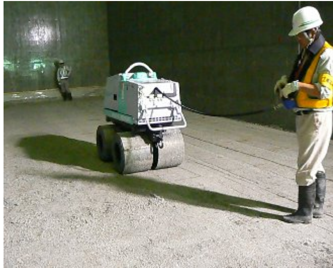
Fig. 9 Compaction by small vibrating roller at side areas
