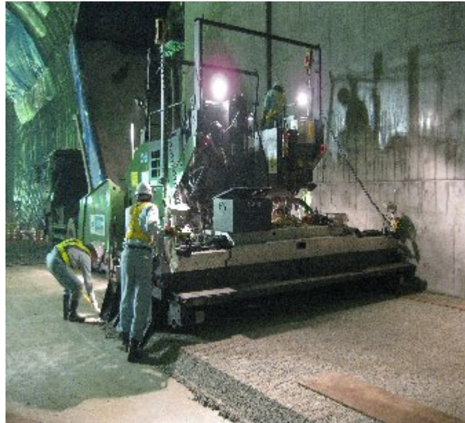
Fig. 7 Spreading by Asphalt Finisher
