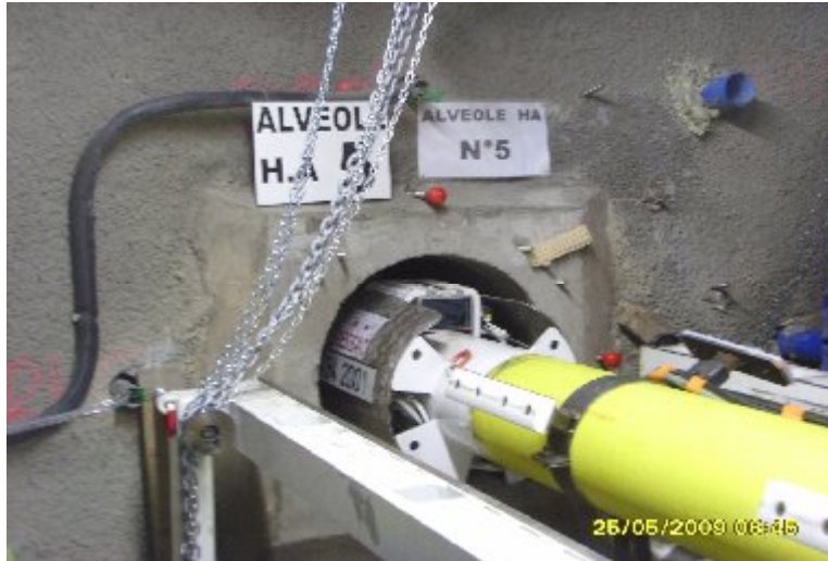
Fig. 11. TBM being introduced into the cell conductor pipe
