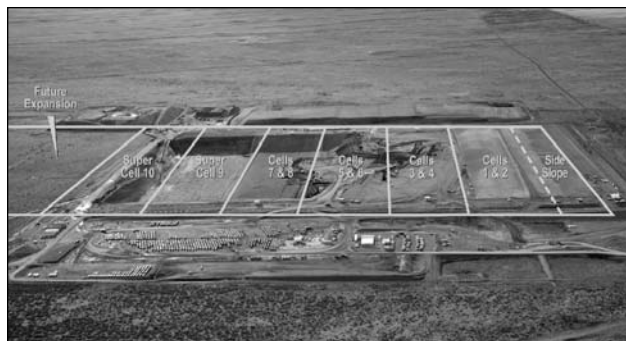
Expansion of Hanford's Environmental Restoration Facility is made possible with funding from the American Recovery and Reinvestment Act. Construction of super cells 9 and 10 will increase waste disposal capacity of the facility by 50 percent and will be completed in September 2011.
