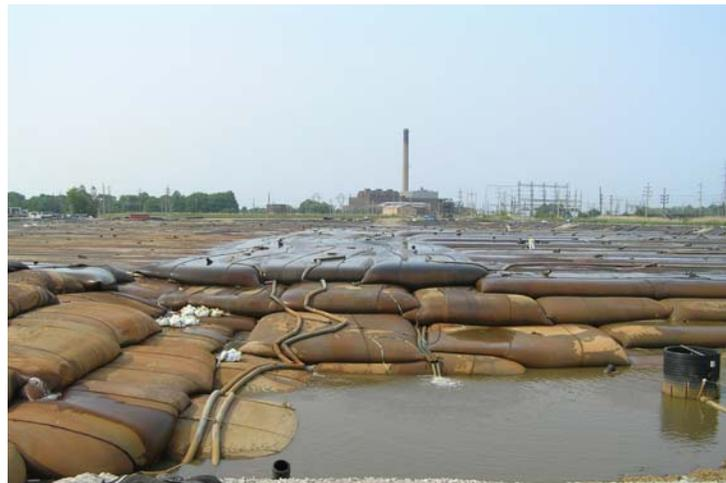
**Fig. 4. The Consolidation Facility showing placement of filled geo-tubes.**
