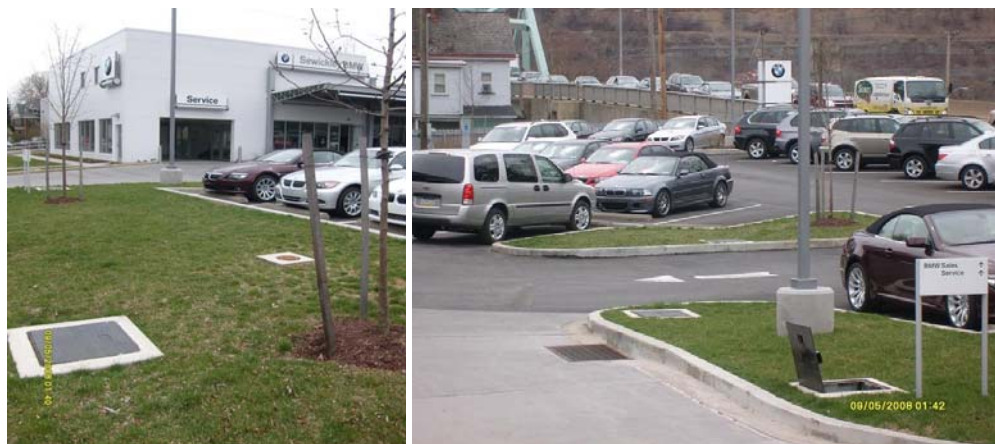
Figure 8. Final Construction Photos of Installed Perozone™ System.
