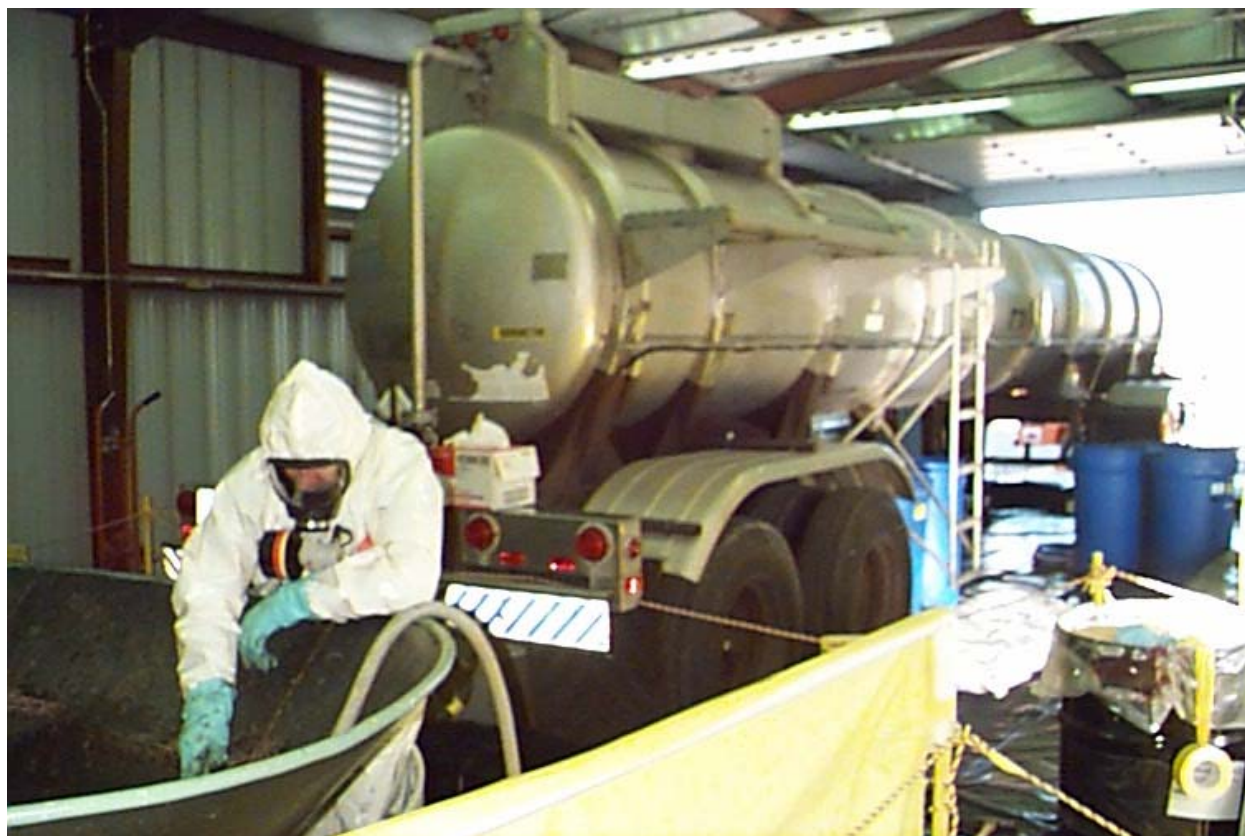
Fig. 1 Pumping septage into tankers for shipment to Perma-Fix for processing.
