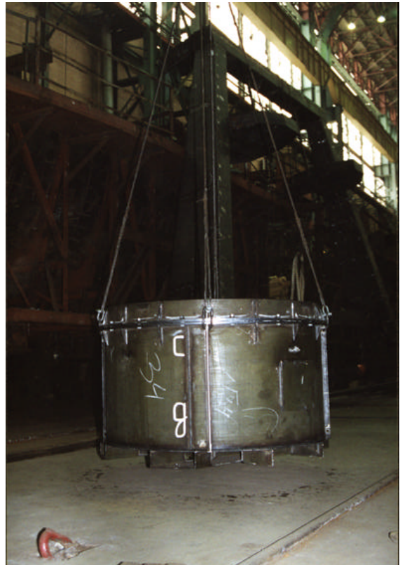
Fig. 2 Steel structure fabrication shop
