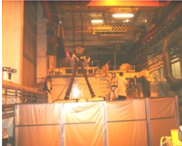
Figure 3: Lifting of Square Steel Support Plate from Cave 9 Roof
